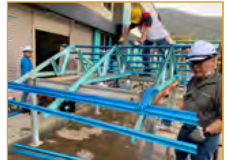
"Roof Truss Installer - RTL1" training conducted by CIDB.
