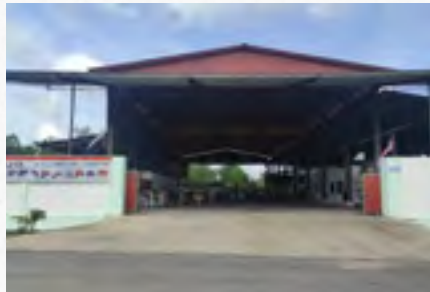
6 Asia Roofing Industries Sdn Bhd Mentakab, Pahang
