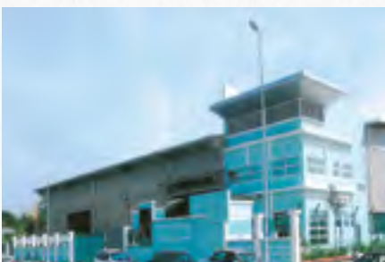
4 Asia Roofing Industries Sdn Bhd Shah Alam, Selangor
