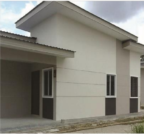
SINGLE-STOREY DETACH House RMR, Kuala Muda
