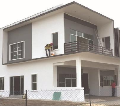
DOUBLE-STOREY TERRACE House, Kuala Terengganu
