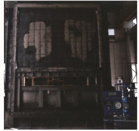
The unexposed face of the wall system after the test
