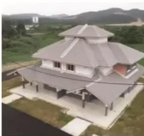
QUARTERS Water Treatment Plant, Semenyih
