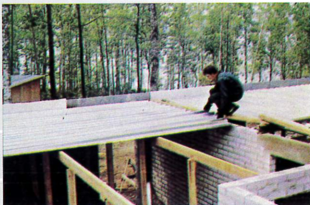
Cut to size steel sheets are easy and quick to assemble. The sparse support cuts down the form expenses
