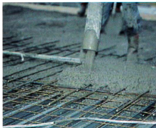
Vibrated concrete pouring on to steel decking reinforced with mesh reinforcement
