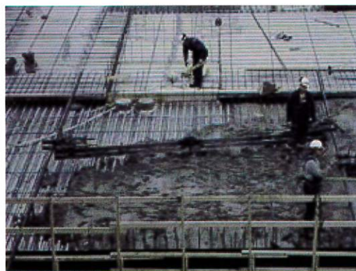
Concreting is on going
