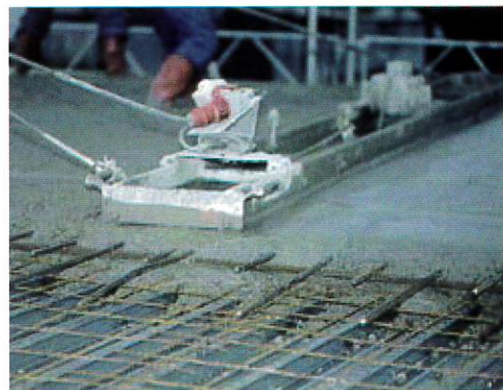
Concreting terminated at opening areas
