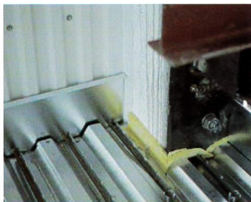
End of sheets are closed with profiled seal to prevent concrete over fend
