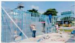
Workers erecting the steel frame wall for Klinik Desa Kempang, Jawa.
