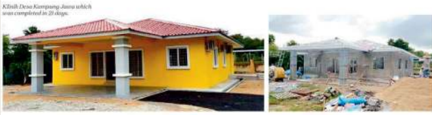
Klinik Desa Kempang, Jawa which was completed in 20 days.
