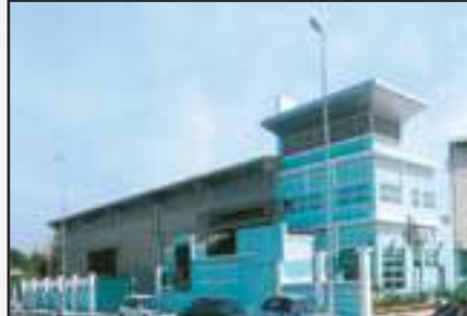
5 Asia Roofing Industries Sdn Bhd Shah Alam, Selangor
