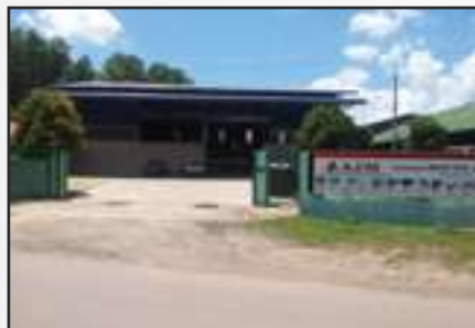
7 Asia Roofing Industries Sdn Bhd Mentakab, Pahang
