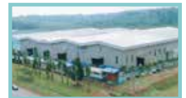
9 ASIA ROOFING INDUSTRIES SDN. BHD. Jalan Seelong, Johor
