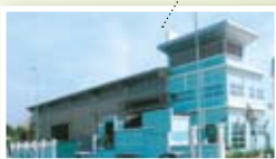
AJIYA SAFETY GLASS SDN BHD Shah Alam, Selangor
