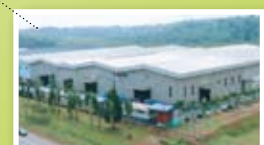
AJIYA SAFETY GLASS SDN. BHD. Segamat, Johor
