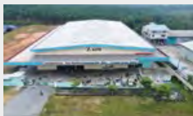
09 Asia Roofing Industries Sdn Bhd Jalan Seelong, Johor
