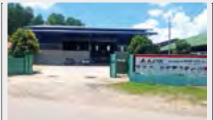
07 Ajiya Roofing Industries Sdn Bhd Mentakab, Pahang
