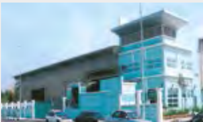
06 Ajiya Safety Glass Sdn Bhd Shah Alam, Selangor
