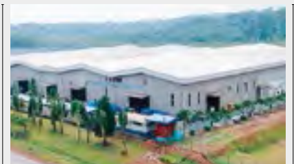
08 Ajiya Safety Glass Sdn Bhd Segamat, Johor.
