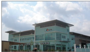
7 Ajiya Safety Glass Sdn Bhd Shah Alam, Selangor
