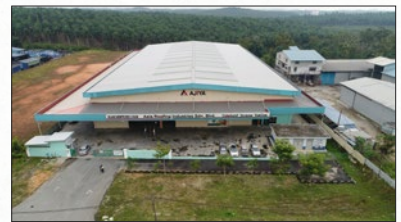
13 Asia Roofing Industries Sdn Bhd Jalan Seelong, Johor
