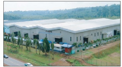
11 Ajiya Safety Glass Sdn Bhd Segamat, Johor
